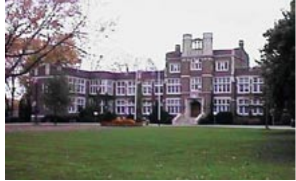
Administration Building, Witney Campus, Ont.
