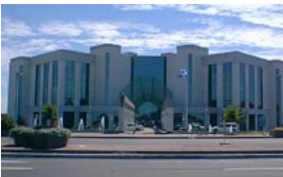
Laval City Provincial Courthouse, Quebec
